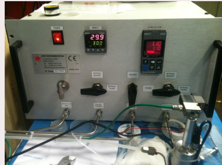
H 2 pressure and low control system
